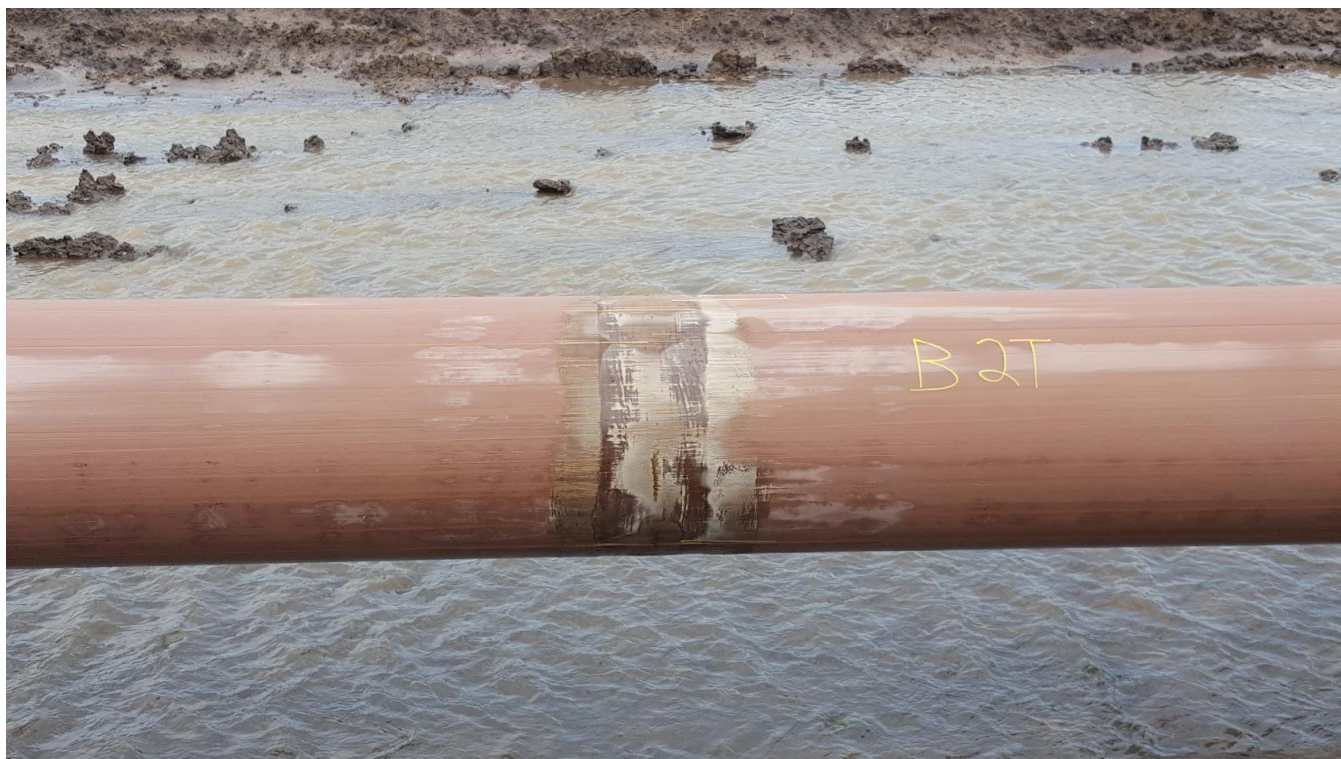
Fig 2. Pipe with ARO showing abrasion wear
