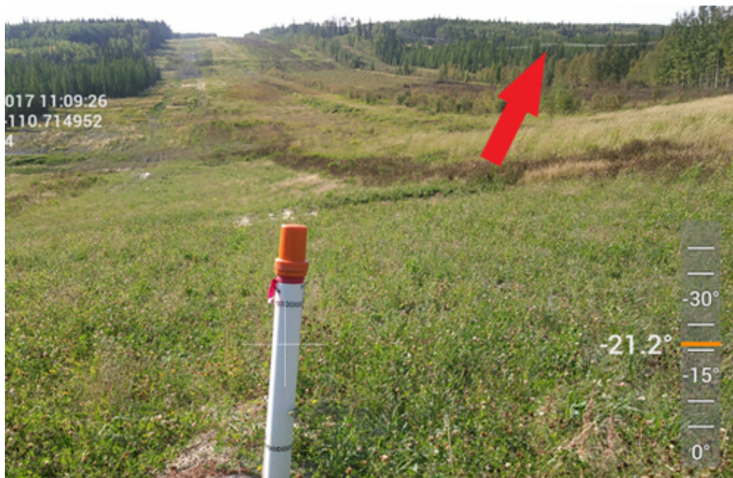
Figure 2: Photo of Missed 240 kV Powerline at KP 82.2
