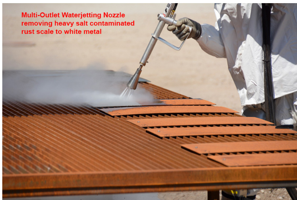
Figure 1: panels being UHP blasted
