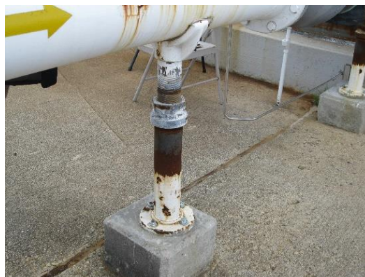
Photo 2. Within an item, there may be sub-items, such as pipe supports, pipe to support interface, and pipe support pedestal.
