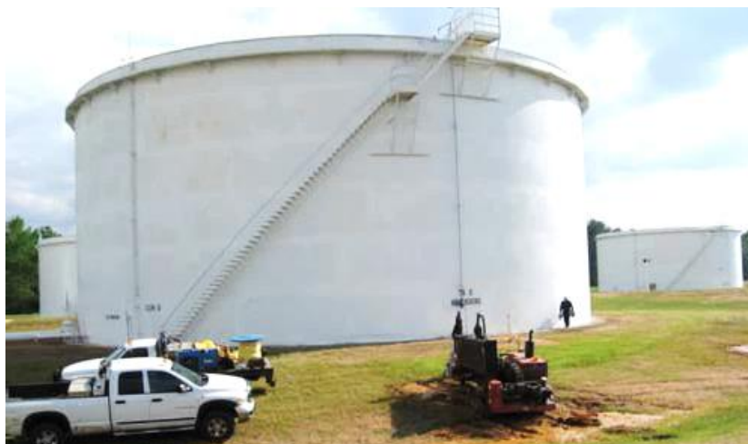
Figure 1: HDD Drilling Below Existing Tank
