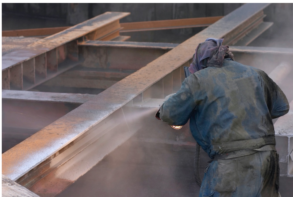
Figure 1. Abrasive blast operator cleaning a steel surface
