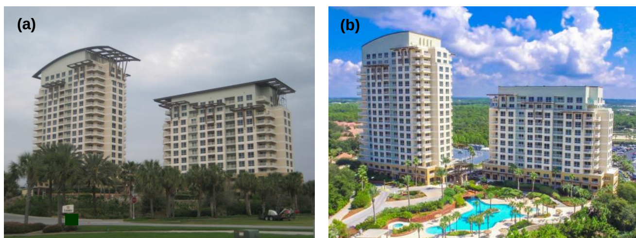
Figure 1. - (a) Towers 1 and 2 with roof canopies (b) Towers with roof canopies removed (1)
