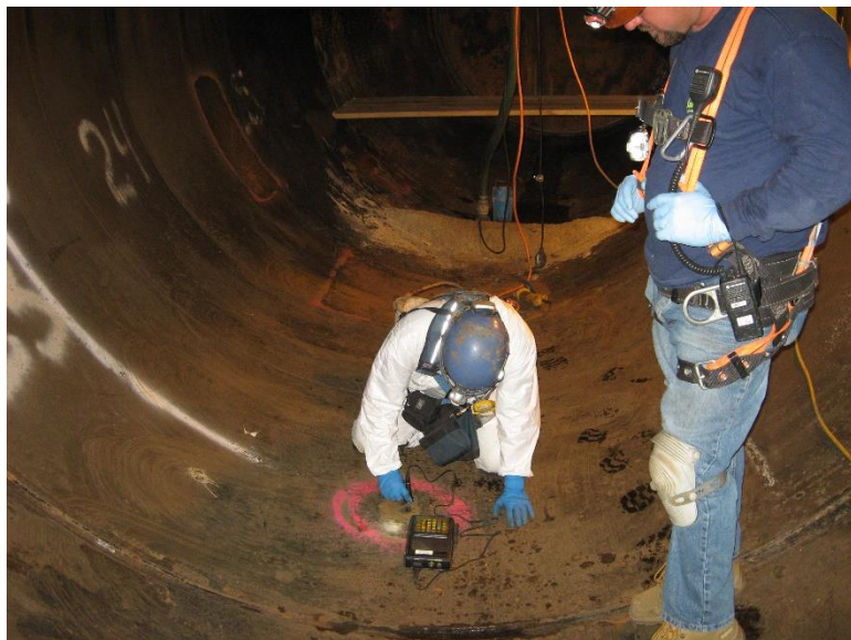
Photo 3. Example of A scan UT testing on a 96-inch diameter pipeline.
