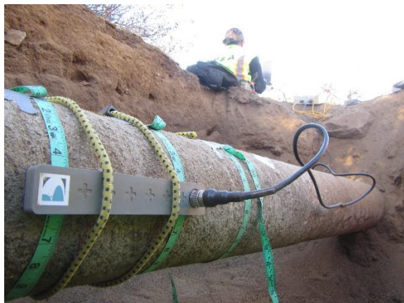
Photo 1. BEM Scanning of mortar-coated metallic pipe.
