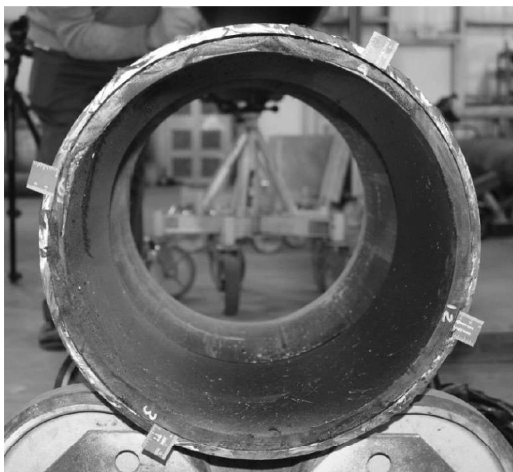
Figure 2: Photo of 16" pipe section typical of polymer lined carbon steel after spec. break. The pipe has a wall thickness ranging 0.312" (7.92 mm) to 3.75" (9.52 mm). The HDPE liner has a wall thickness of approximately 0.5" (12.7 mm).
