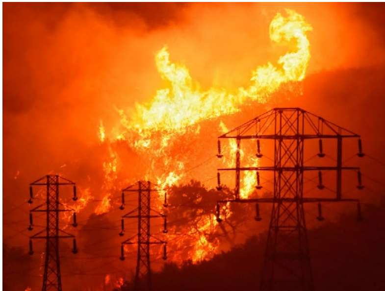
Figure 1: Wildfire Approaching Close to Power Transmission Structures (Mike Eliason/AP)
