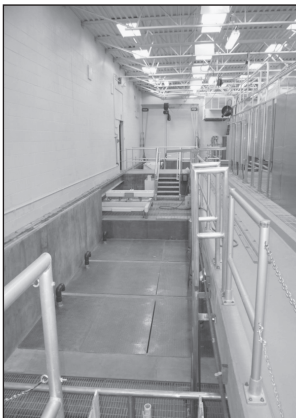
Figure 4.2-3 Submerged Membrane Tanks With Jib Crane Tracks and Control Cabinets at the Marys Lake Water Treatment Plant
