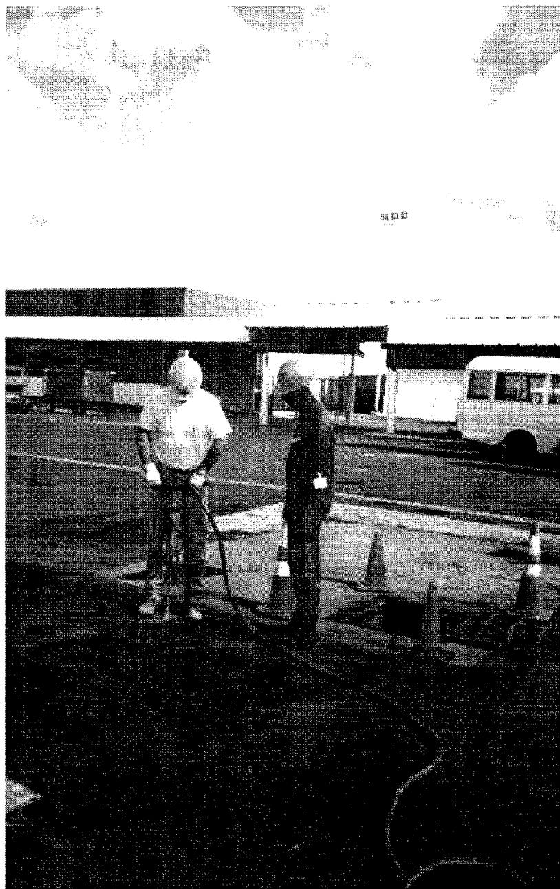
Figure 8. Drilling to Install Tracer Ports
