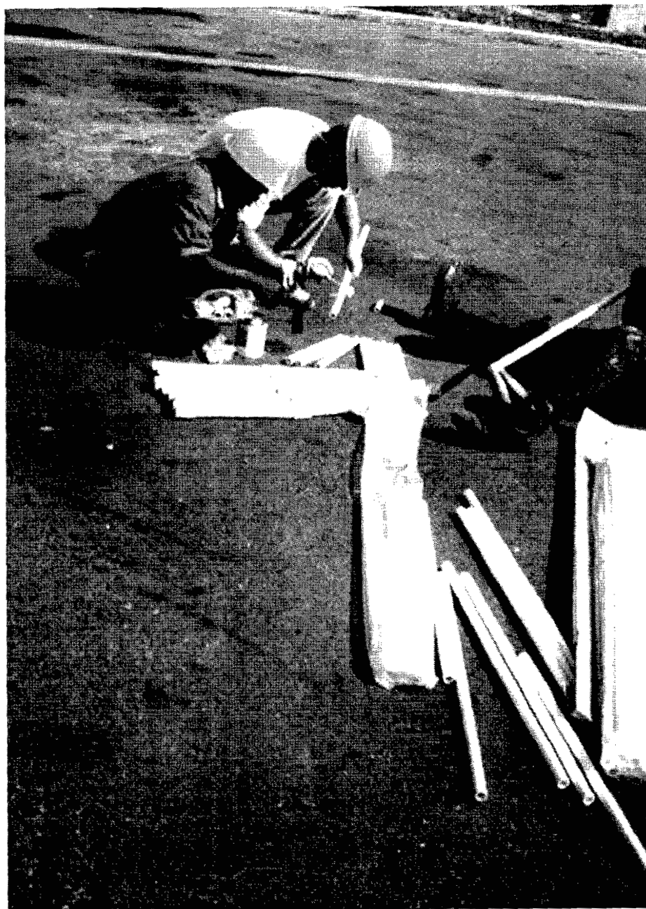
Figure 10. Installing Sampling Ports for Tracer
