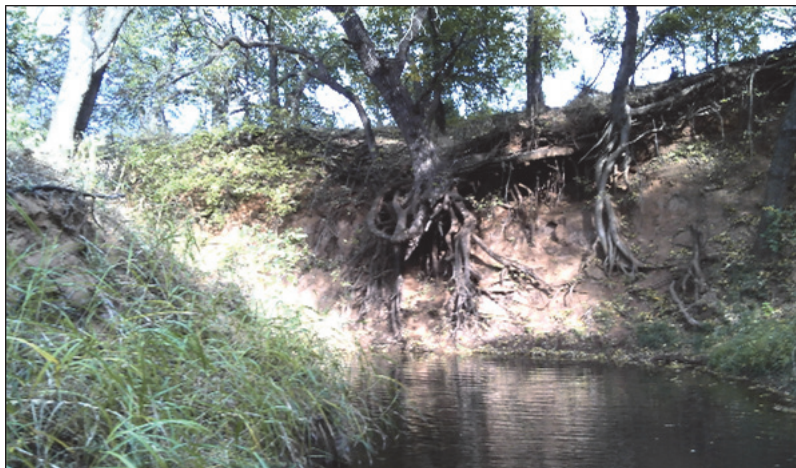
Figure 10—Example of Bank Erosion as a Source of In-channel Woody Debris
