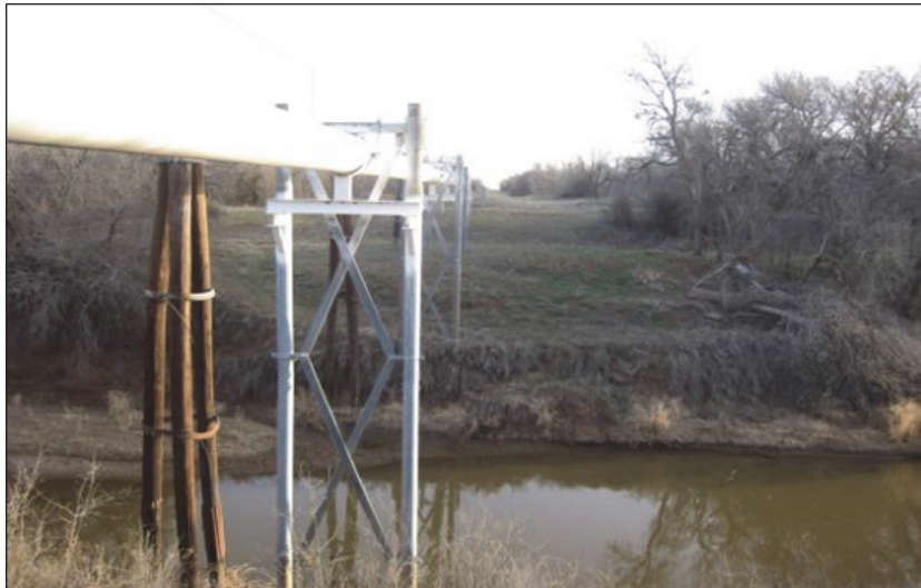
Figure 13—Example of Engineered Span Supported by H-braces
