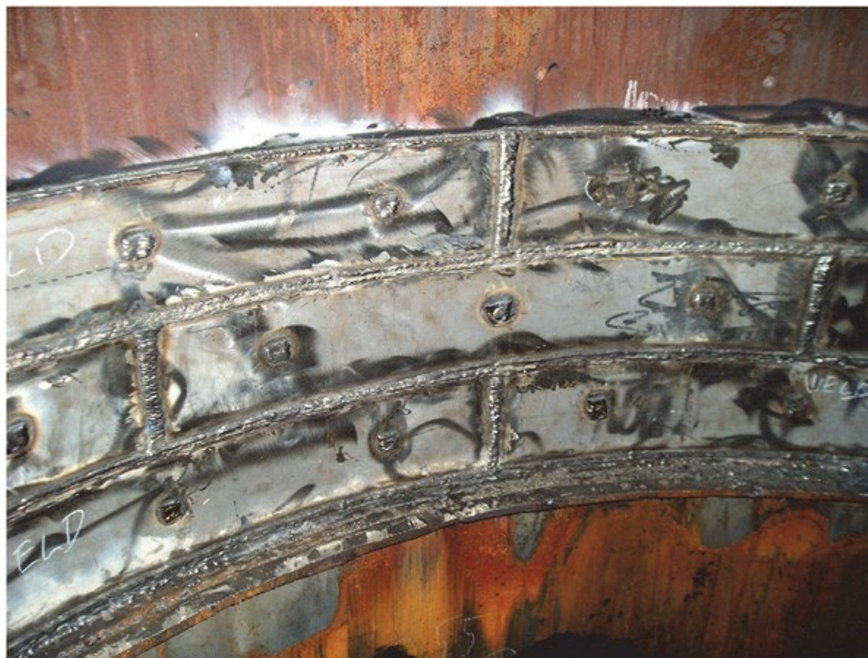
Figure 13—Strip-lined Vessel
