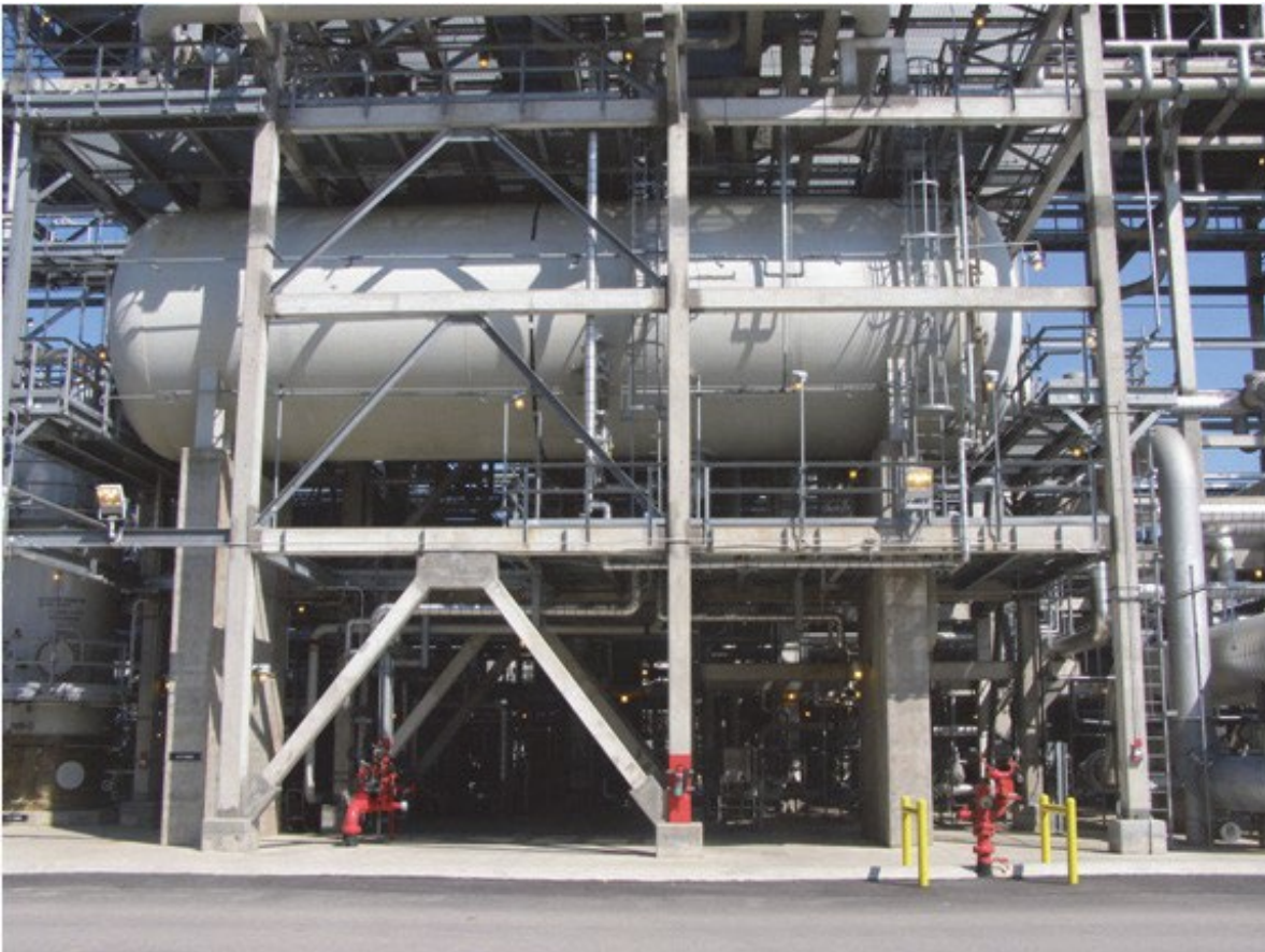
Figure 11—Horizontal Vessel
