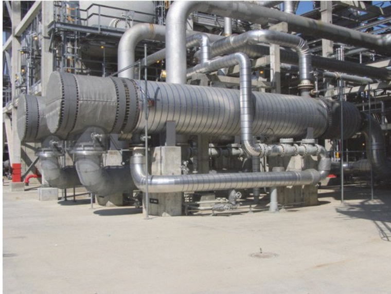
Figure 7—Example of a Horizontal Heat Exchanger
