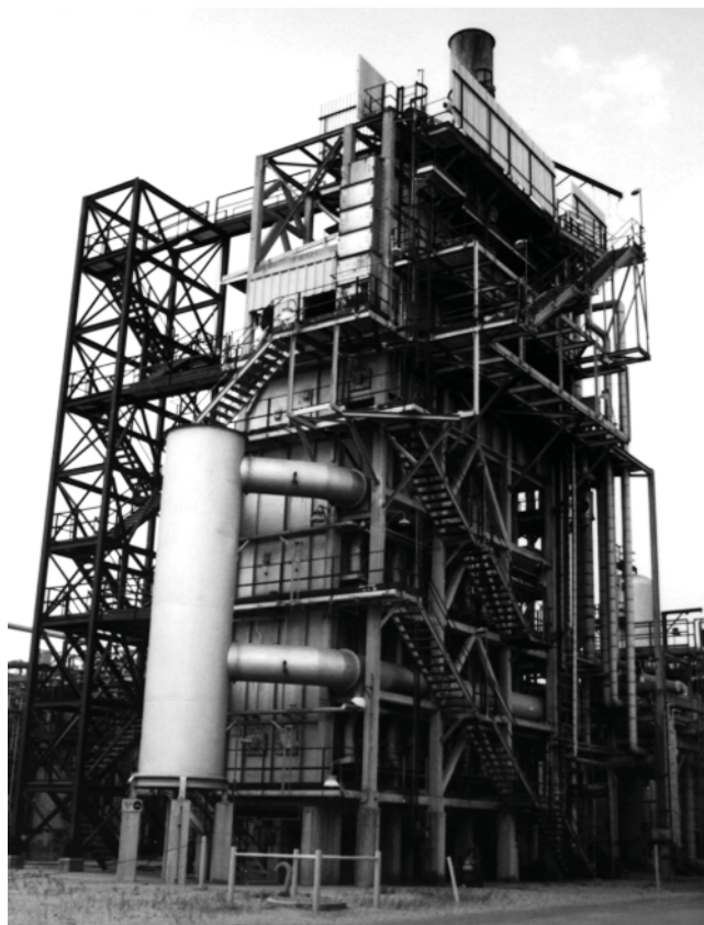
Figure 3—One Type of Steam-Methane Reforming Furnace
