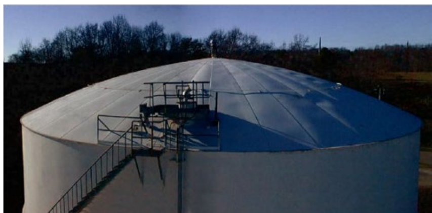
Figure 3—Umbrella Roof Tank
