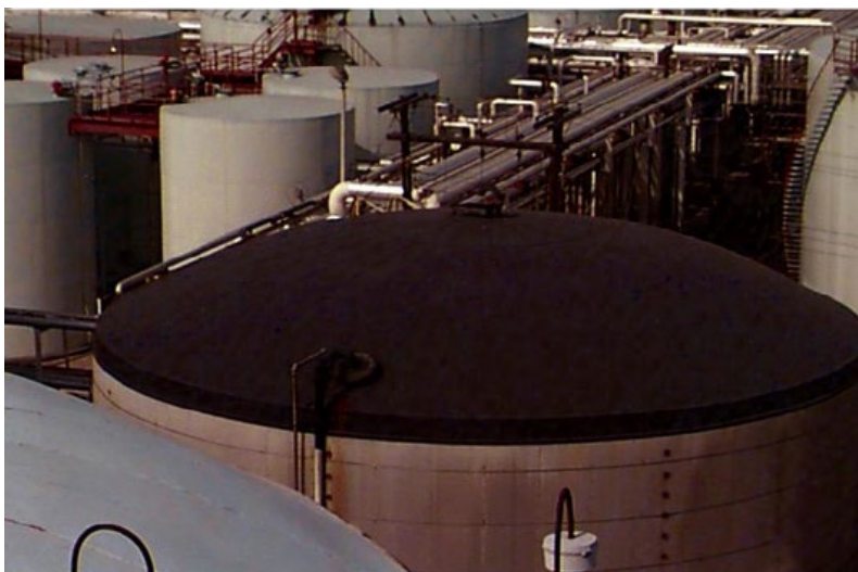
Figure 2—Self-supporting Dome Roof Tank
