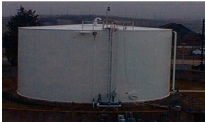
Figure 1—Fixed Cone Roof Tank
