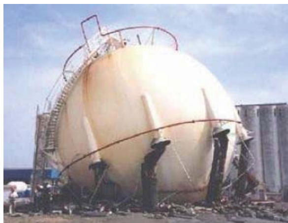
Figure 5—Failure of Sphere Legs Due to CUF
