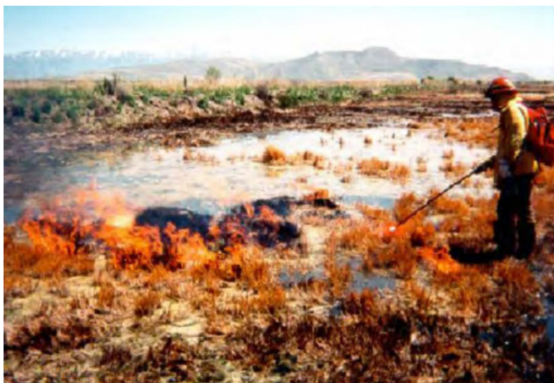
Figure 7—Igniting Oil with a Propane Burner (Photo source: API, 2002)
