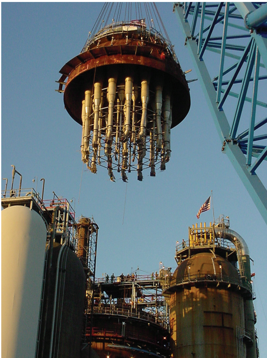
Figure 2—Replacement of Primary (Outer Ring) and Secondary (Inner Ring) Cyclones
