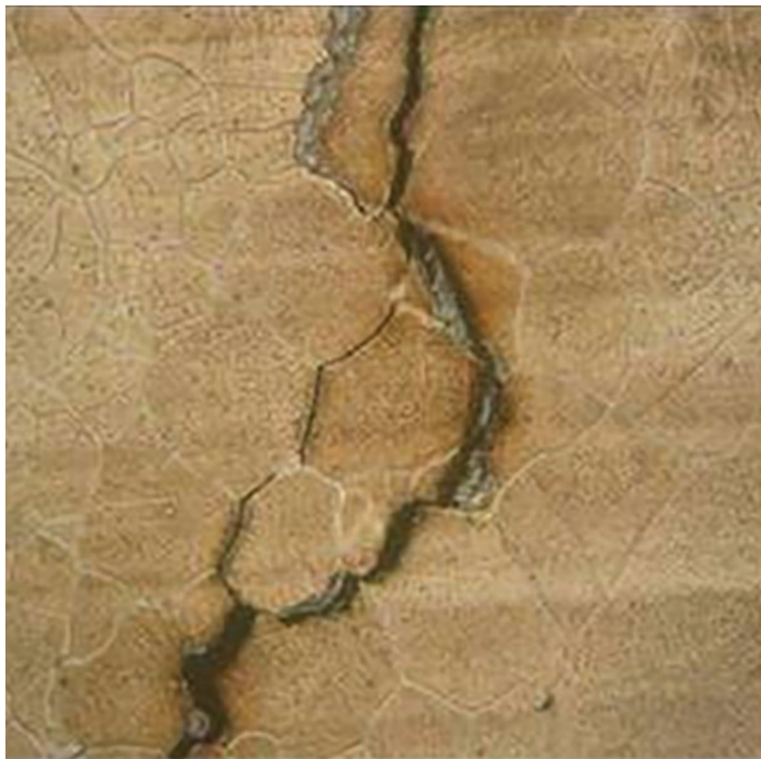
Figure 13—Cross Section of a Crack at the Toe of One of the TC Shields Showing Intergranular SRC
