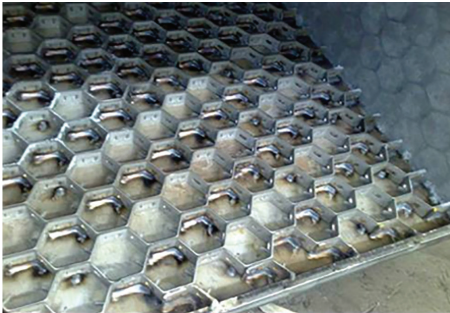
Figure 3—Example of New Hexagonal Mesh Welded Inside a Regenerator Cyclone
