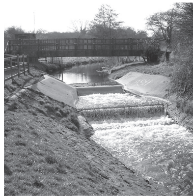
b) Trapezoidal-throated flume
