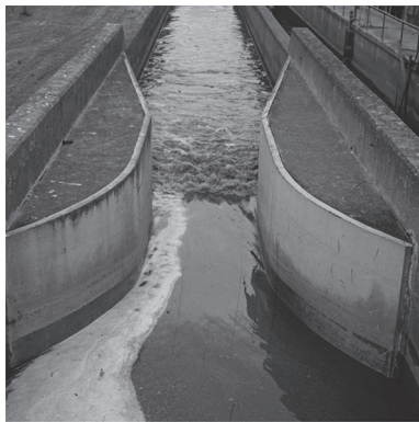
a) Rectangular-throated flume
