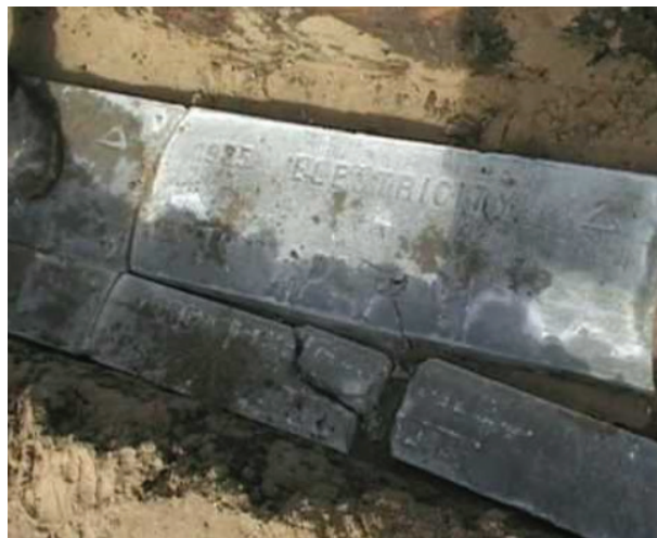
Figure 2 — Brick protection over utility
