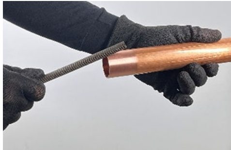
FIG. 3 Remove Any Burrs on the Outside of the Tube Ends
