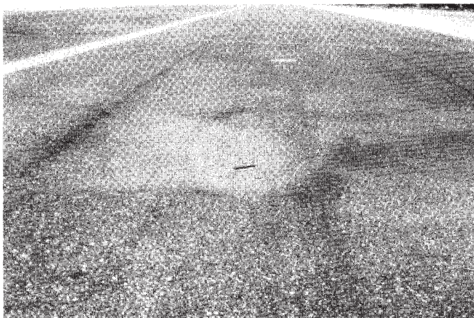
FIG. X1.26 Medium-Severity Depression
