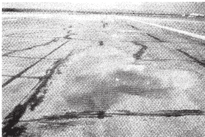
FIG. X1.27 High-Severity Depression (2 in. (50 mm))
