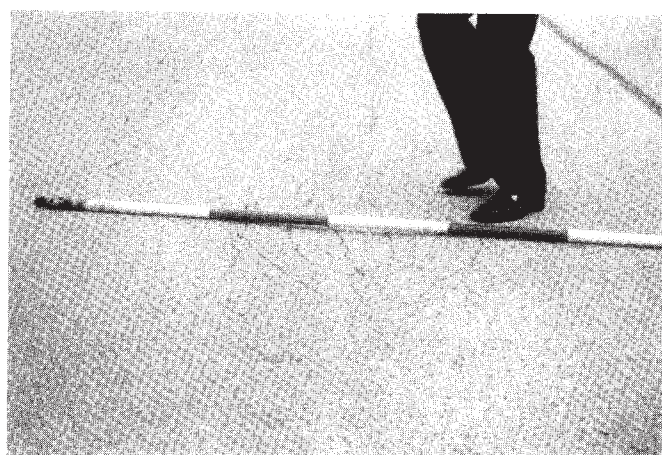
FIG. X1.4 Medium-Severity Alligator Cracking (Note the Depression Occurring with the Cracking)
