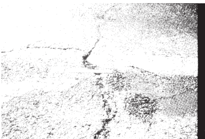
FIG. X1.42 High-Severity Longitudinal Crack
