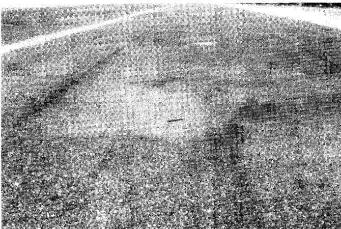
FIG. X1.26 Medium-Severity Depression
