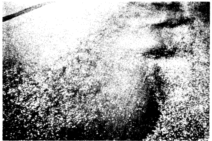
FIG. X1.23 High-Severity Corrugation
