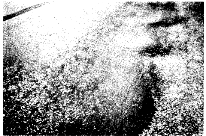
FIG. X1.23 High-Severity Corrugation
