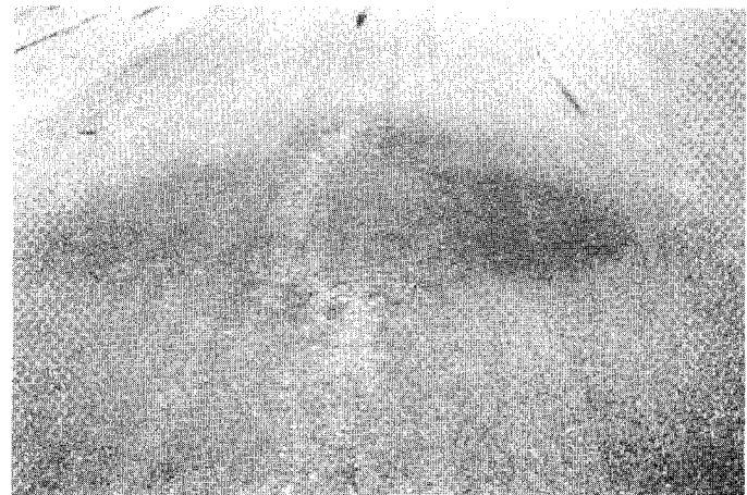
FIG. X1.24 Low-Severity Depression
