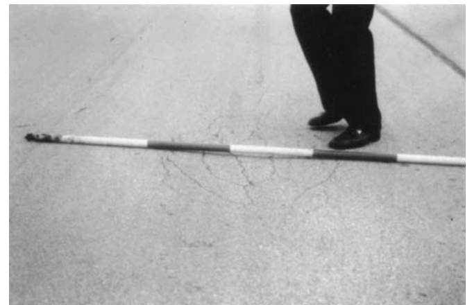
FIG. X1.4 Medium-Severity Alligator Cracking (Note the Depression Occurring with the Cracking)
