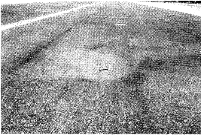
FIG. X1.26 Medium-Severity Depression
