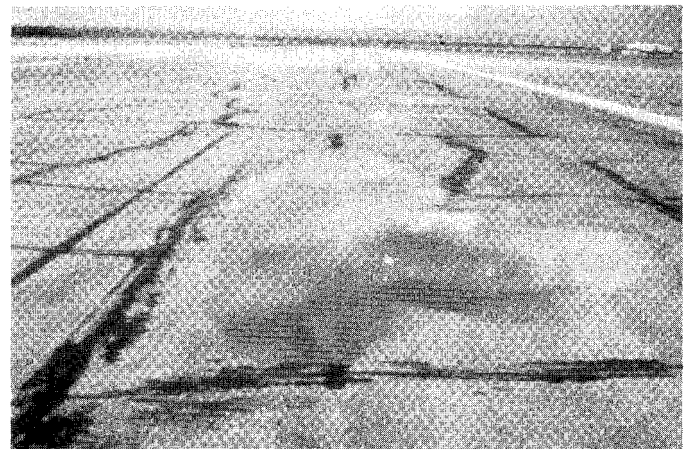
FIG. X1.27 High-Severity Depression (2 in. (50 mm))
