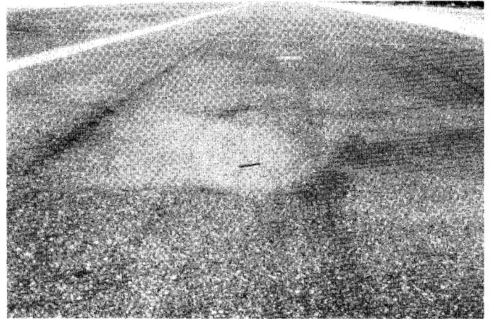
FIG. X1.26 Medium-Severity Depression
