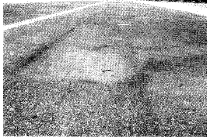
FIG. X1.26 Medium-Severity Depression
