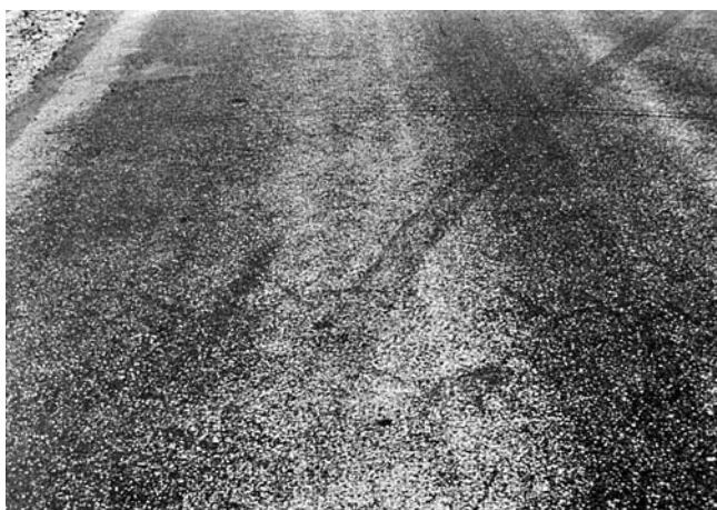
FIG. X1.4 Low-Severity Bleeding
