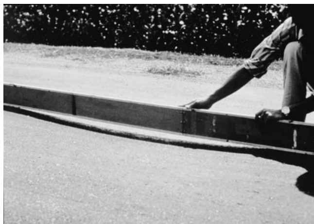
FIG. X1.17 Medium-Severity Depression
