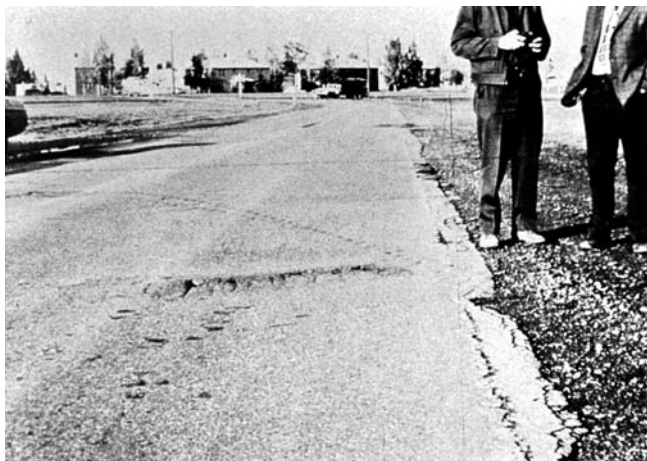
FIG. X1.11 Medium-Severity Bumps and Sags
