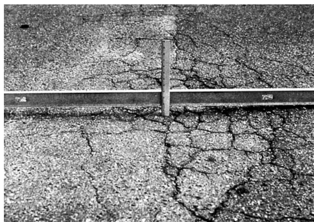
FIG. X1.18 High-Severity Depression
