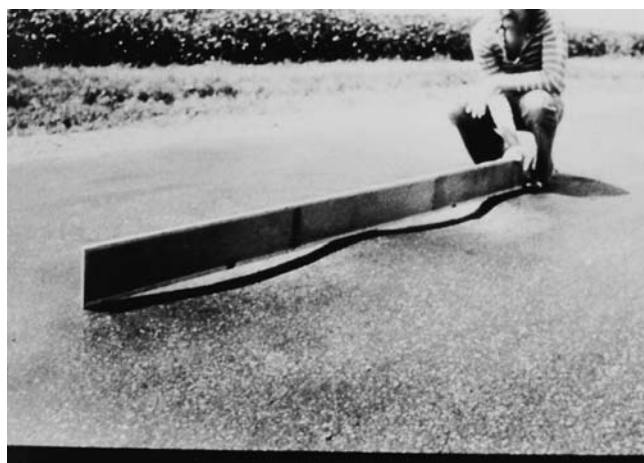
FIG. X1.15 High-Severity Corrugation
