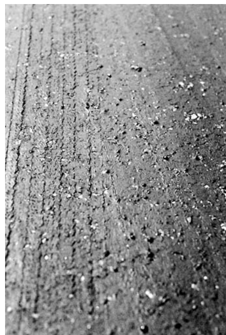
FIG. X1.6 High-Severity Bleeding
