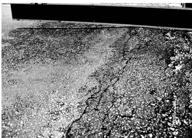
FIG. X1.12 High-Severity Bumps and Sags
