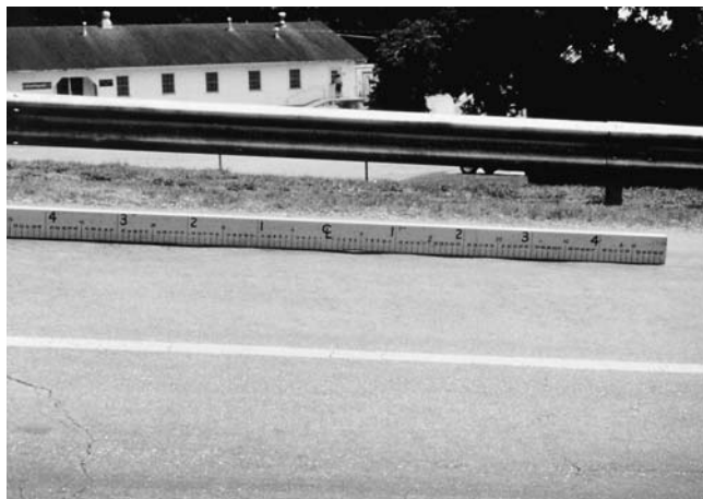
FIG. X1.13 Low-Severity Corrugation
