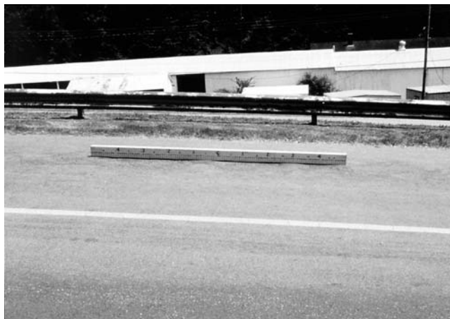
FIG. X1.14 Medium-Severity Corrugation
