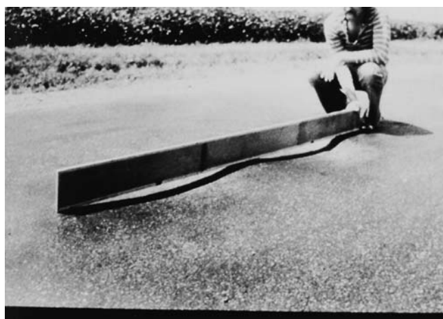
FIG. X1.15 High-Severity Corrugation
