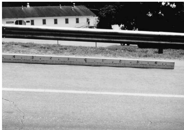
FIG. X1.13 Low-Severity Corrugation
