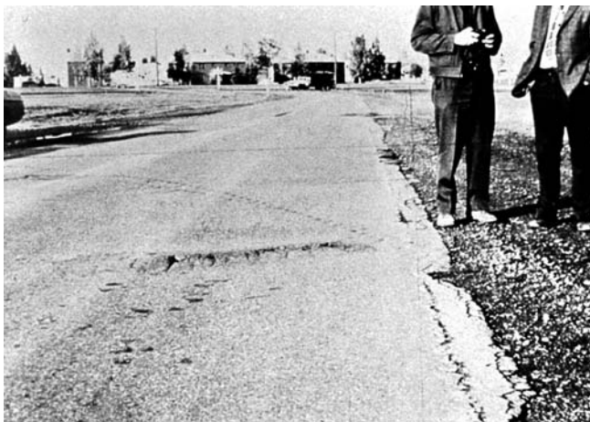
FIG. X1.11 Medium-Severity Bumps and Sags
