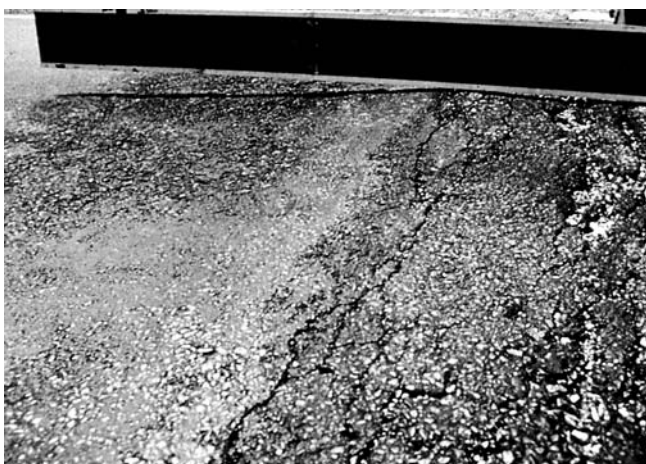
FIG. X1.12 High-Severity Bumps and Sags
