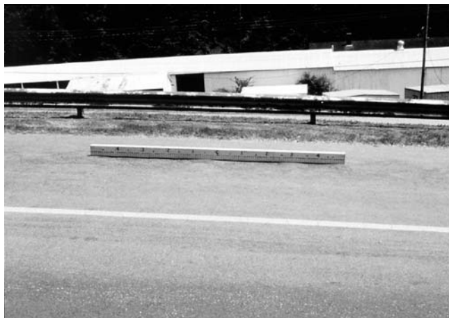
FIG. X1.14 Medium-Severity Corrugation
