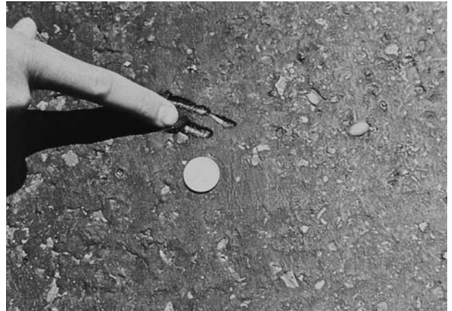
FIG. X1.5 Medium-Severity Bleeding
