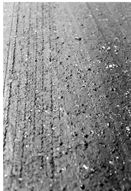
FIG. X1.6 High-Severity Bleeding
