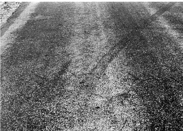
FIG. X1.4 Low-Severity Bleeding
