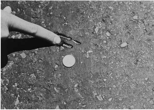
FIG. X1.5 Medium-Severity Bleeding
