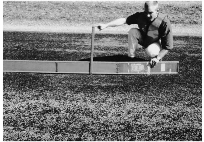
FIG. X1.16 Low-Severity Depression
