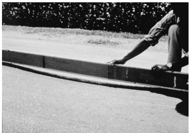
FIG. X1.17 Medium-Severity Depression
