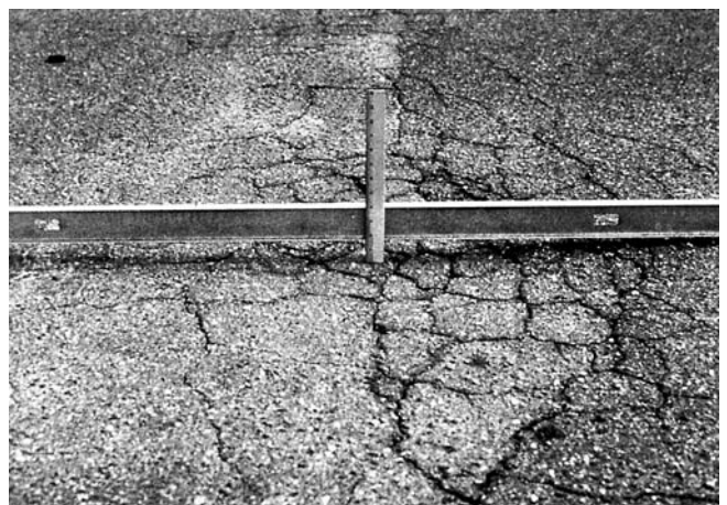
FIG. X1.18 High-Severity Depression
