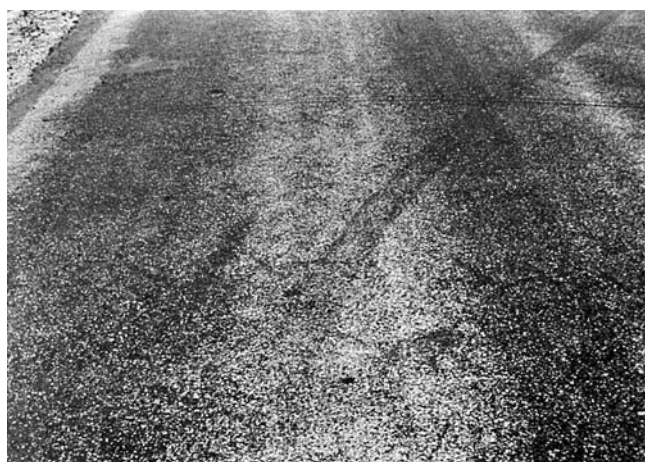
FIG. X1.4 Low-Severity Bleeding
