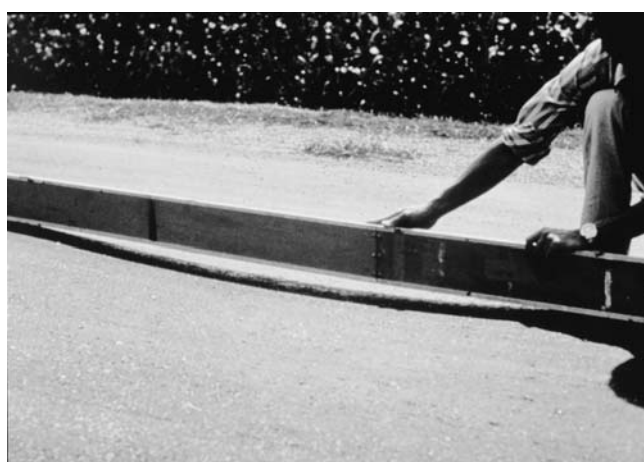
FIG. X1.17 Medium-Severity Depression
