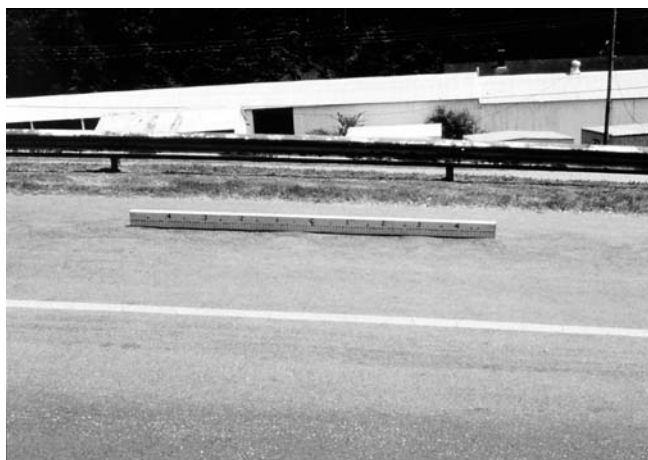
FIG. X1.14 Medium-Severity Corrugation
