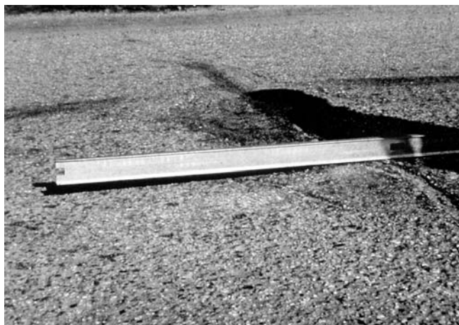
FIG. X1.10 Low-Severity Bumps and Sags
