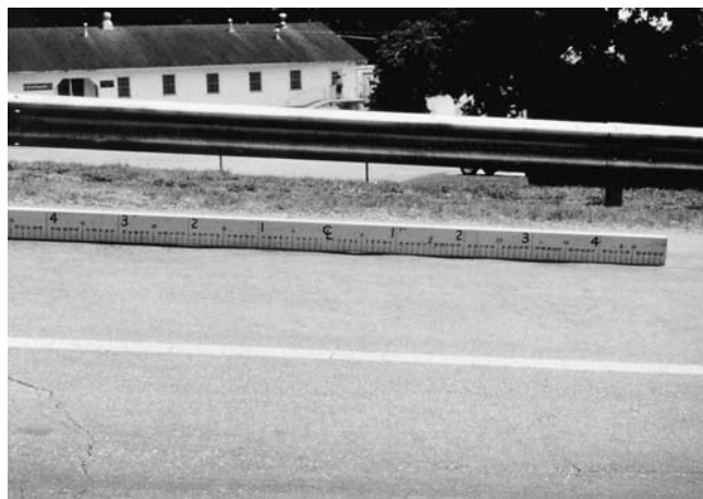
FIG. X1.13 Low-Severity Corrugation
