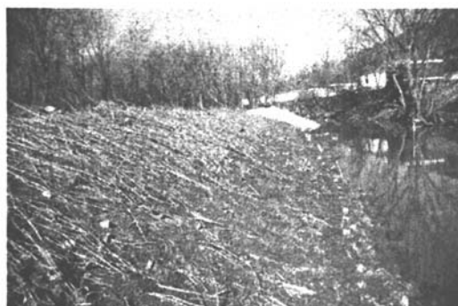
FIG. 1 Brushmattress after Light Backfill of Soil
