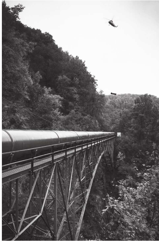
Figure 1-1 Steel pipe penstock on bridge
