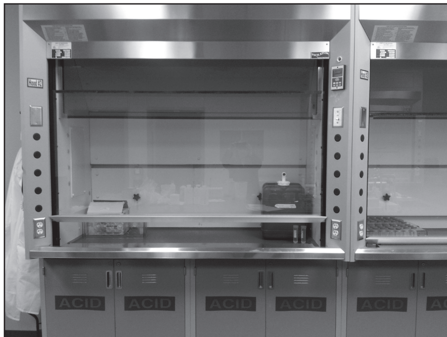
Figure 1-7 Safe storage and labeling for fume hood
