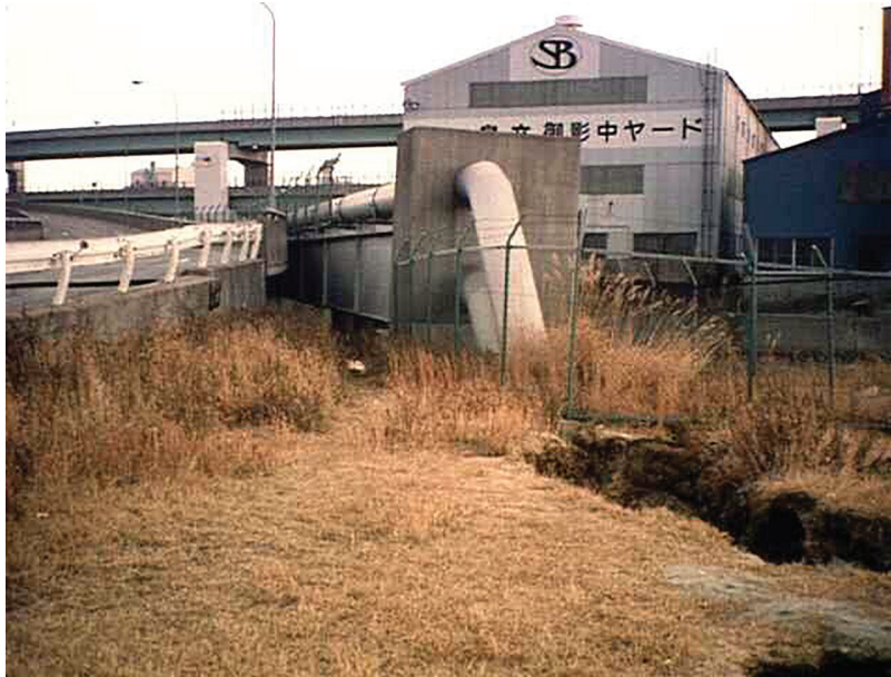
Figure 2-5A Ground crack resulting from lateral spreading in Kobe, Japan in 1995
