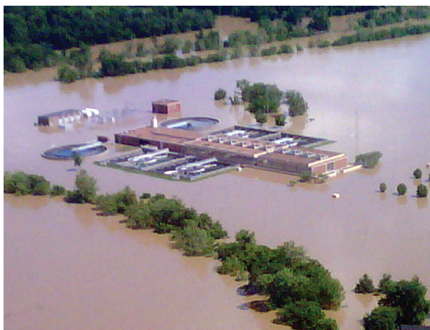
Figure 2-6 Flooded K.R. Harrington Water Treatment Plant in Nashville
