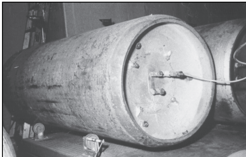
Figure 4-6 Ton containers stored on trunnions
