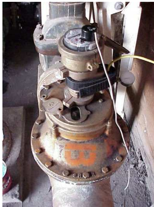
Figure 3-4 Compound adapter and sensor
