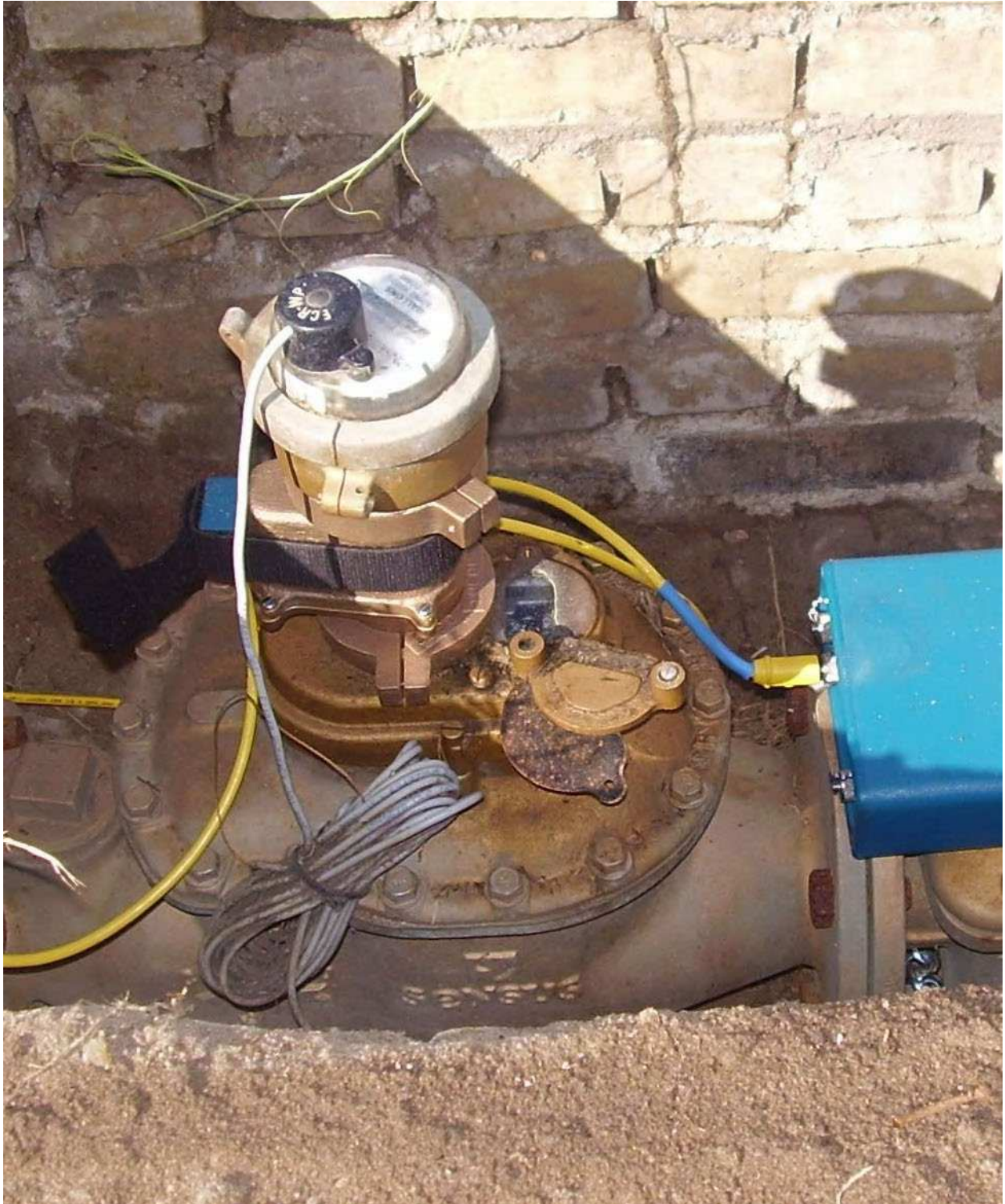
Figure 3-5 Recording demand profiles from large compound meters may require an adapter.
