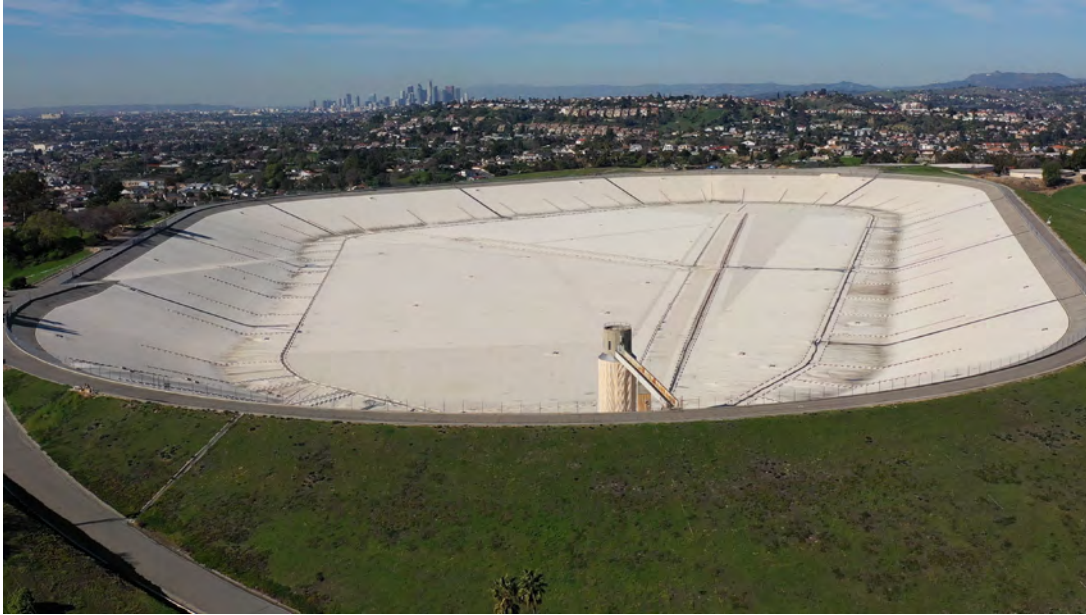
Figure 2-1 Floating cover and geomembrane liner installed in 1998 on 525-mil-gal potable water reservoir in Monterey Park, Calif.
