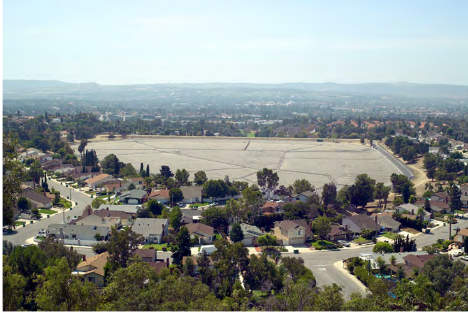
Figure 2-3 Floating cover and geomembrane liner installed in 2001 on 275-mil-gal potable water reservoir in Mission Viejo, Calif.
