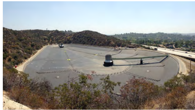
Figure 2-4 Floating cover installed in 2014 on 83-mil-gal potable water reservoir in Eagle Rock, Calif.
