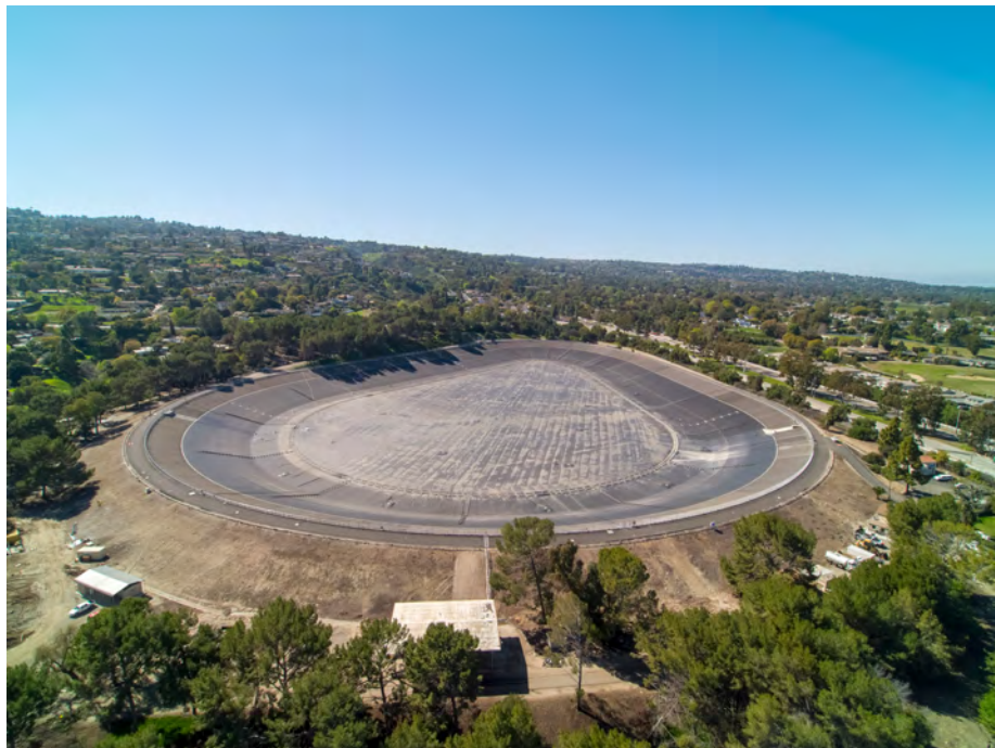
Figure 2-2 Floating cover and geomembrane liner installed in 2017 on 360-mil-gal potable water reservoir in Rolling Hills Estates, Calif.
