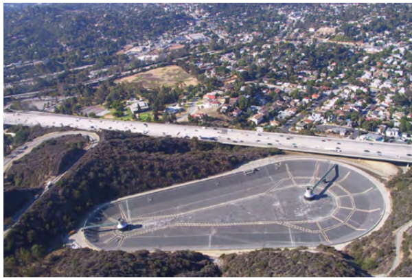
Figure 2-4 Floating cover installed in 2014 on 83-mil-gal potable water reservoir in Eagle Rock, Calif.
