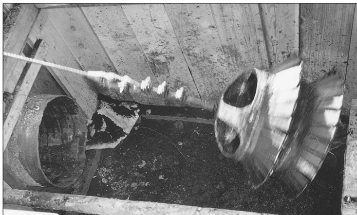
Figure 4-1 Drag cleaning, in which a winch pulls a mechanical cleaner through the pipe
