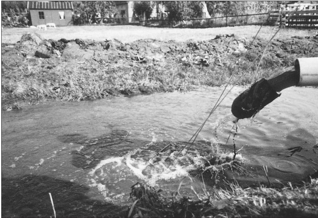
Figure 4-4 Loose debris flushed ahead of the pig
