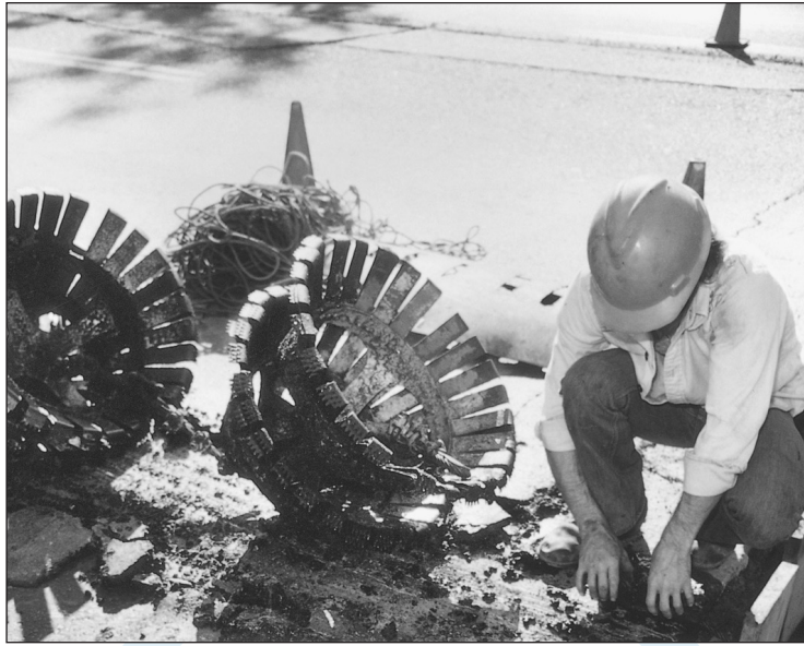
Figure 4-7 Several scraper units assembled together in the field
