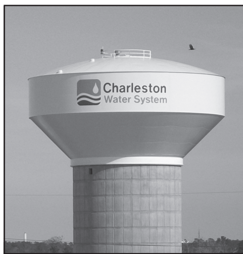
Figure 1-26 Composite elevated welded tank
