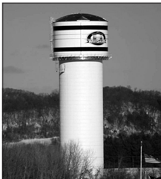
Figure 1-28 Composite elevated bolted tank
