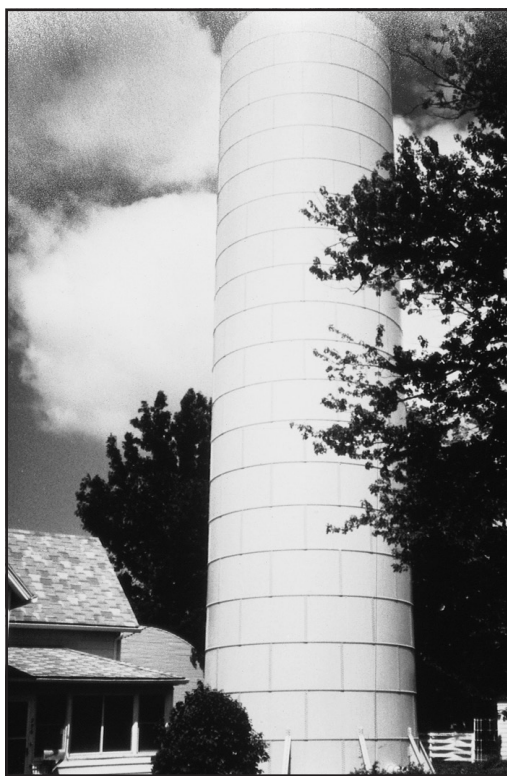
Figure F-1 A tank constructed in 1902 is still serving Wabash, Ind., with practically no metal loss
