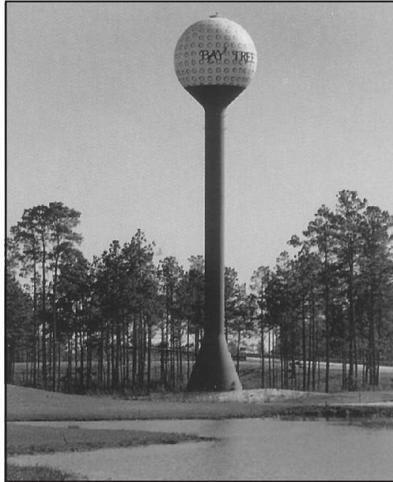
Figure 1-19 Spherical single-pedestal tanks give pleasant silhouette
