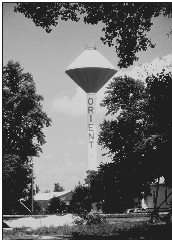
Figure 1-21 Alternative single-pedestal tank design
