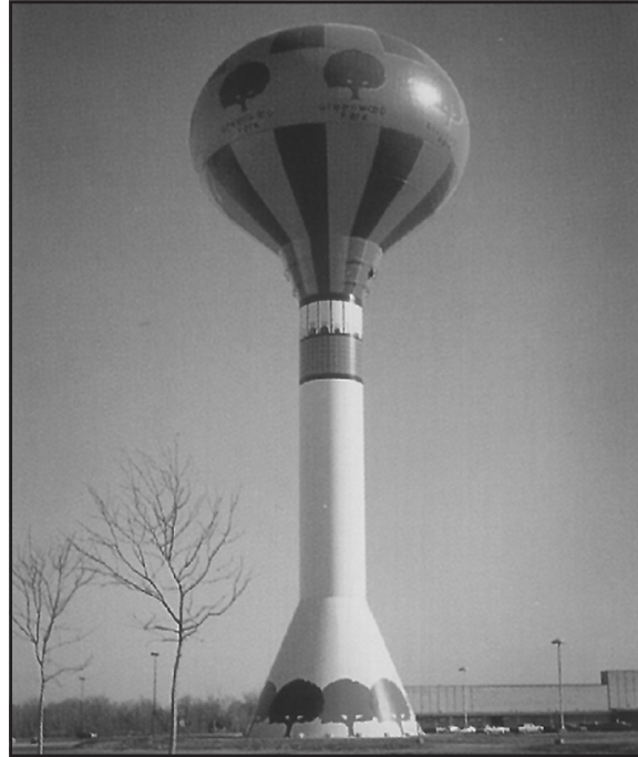
Figure 1-22 Large-capacity single-pedestal elevated tank
