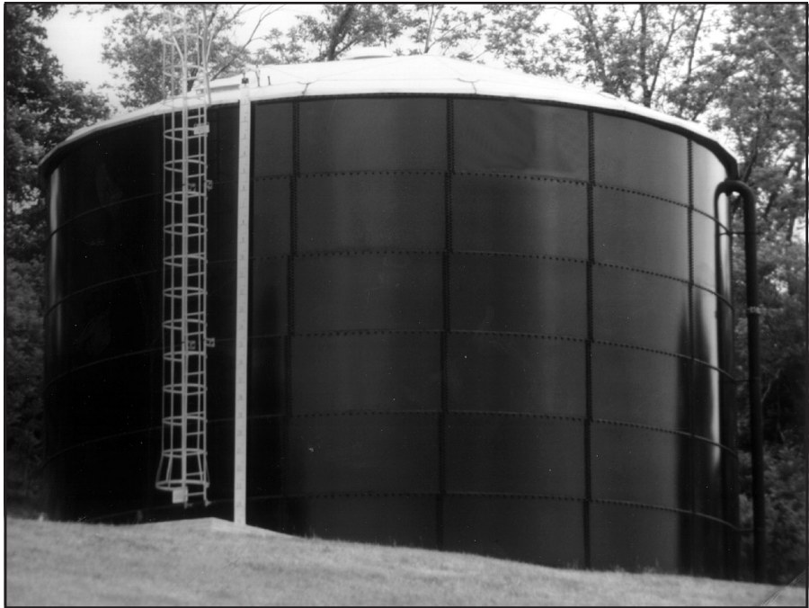
Figure 1-3 Bolted steel reservoir, glass fused to steel
