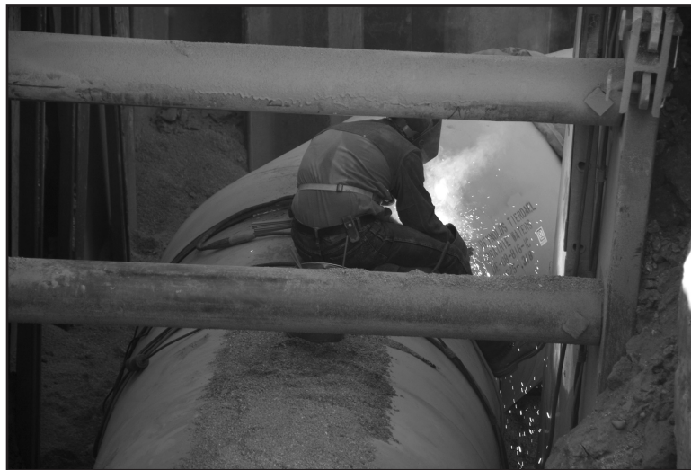
Figure 3-3 Pipeline repair
