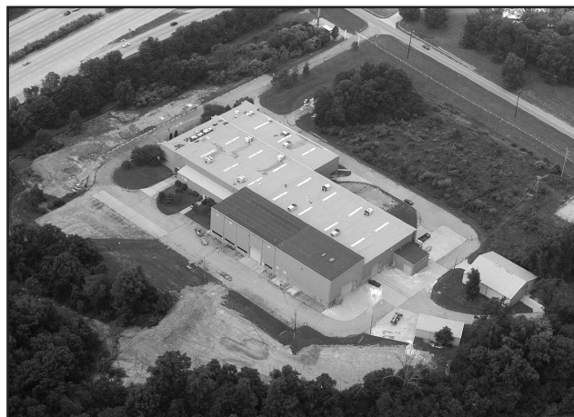
Figure I-4 Headquarters/admin building (courtesy of A. Kramer)
