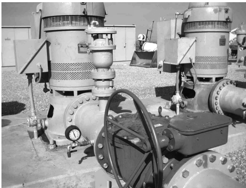
Figure 1-2 An air valve installed on the outlet of a pump and upstream of the check valve
