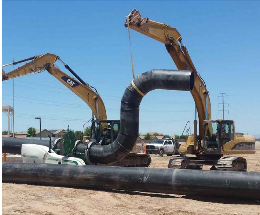
Figure 2-4 Prefabricated 90° elbow being attached in field
