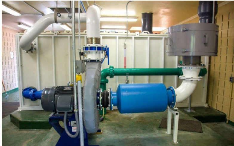
Figure 2-10 A centrifugal blower
