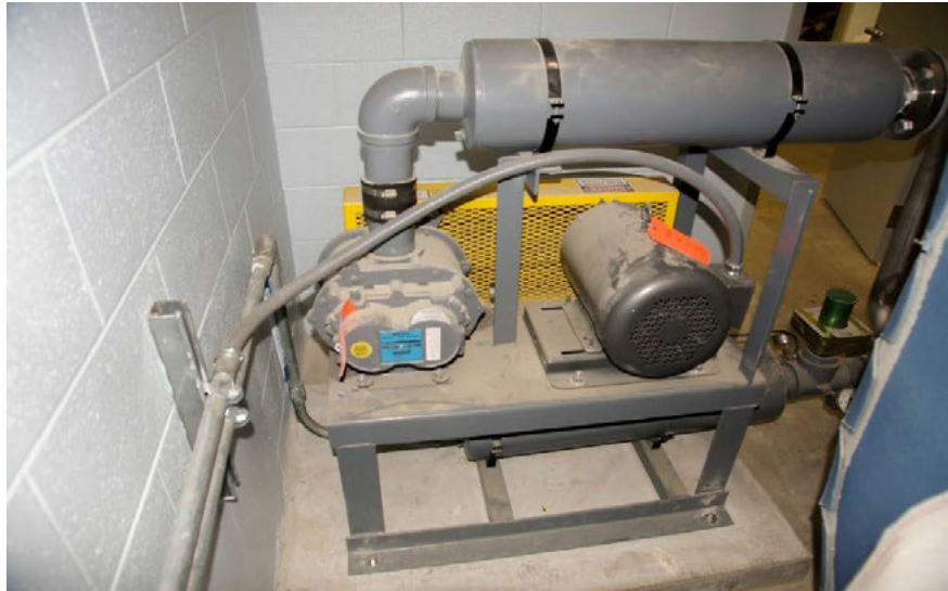
Figure 2-12 A positive displacement-type blower
