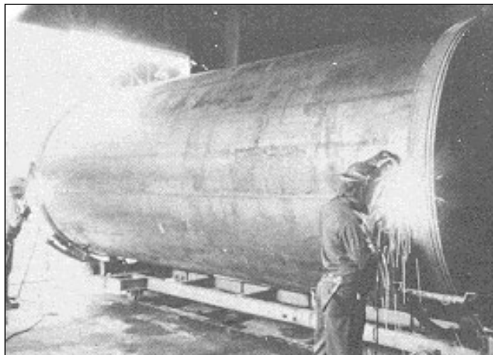
Figure 2-4 Welding joint rings to cylinder
