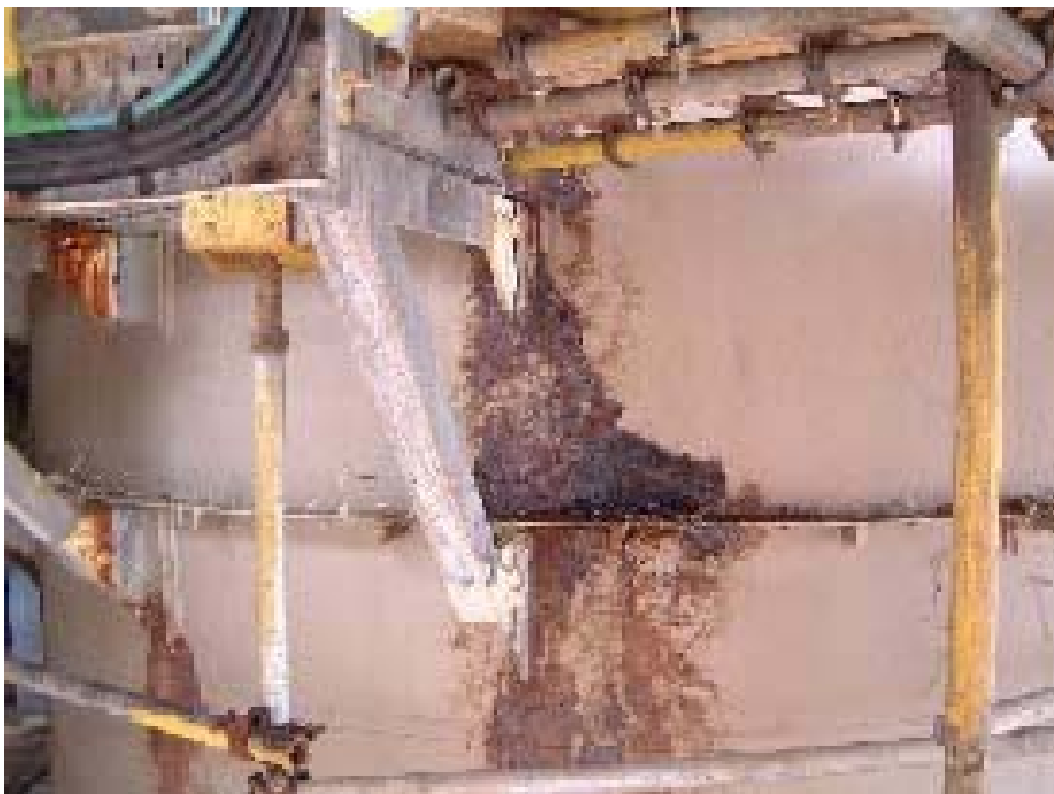
Figure 1 - Designs/layout which are difficult to insulate
