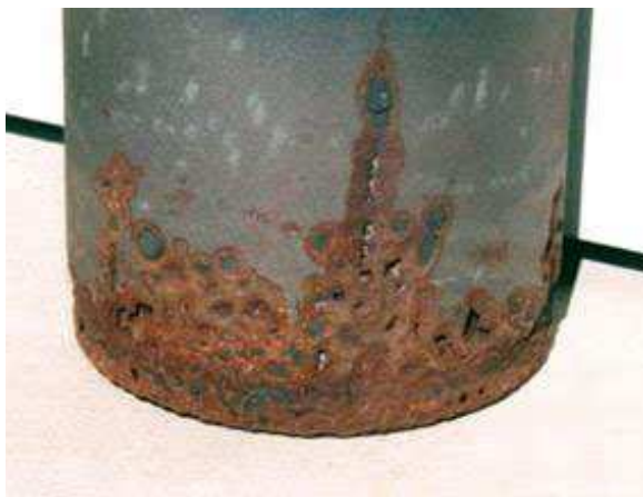
Figure 3—General corrosion with pitting
