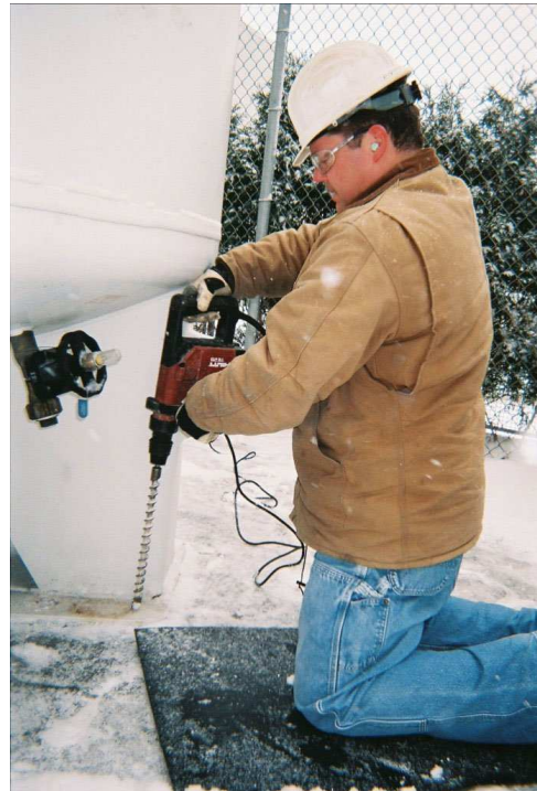
Employee using rotary hammer drill
