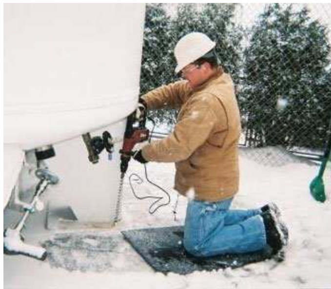
Employee using kneeling pad while repairing equipment
